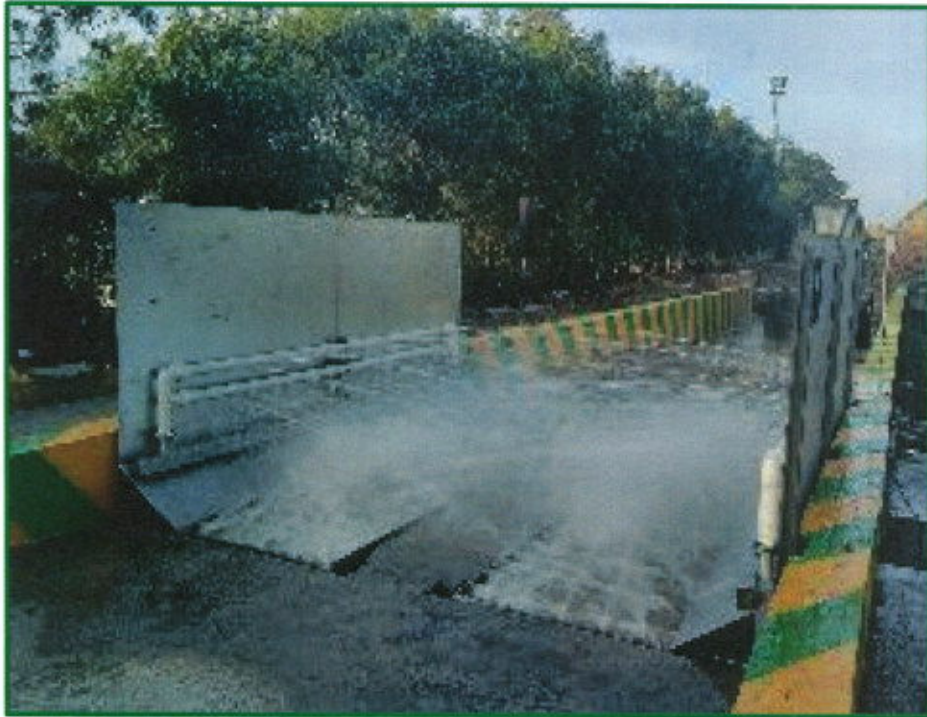
Automatic Tyre Washer at Weigh bridge
